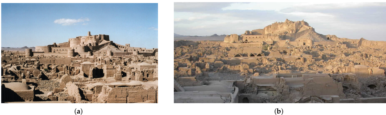
Figure 7. Bam citadel; (a) before the 2003 Earthquake; (b) after the earthquake (UNESCO).
