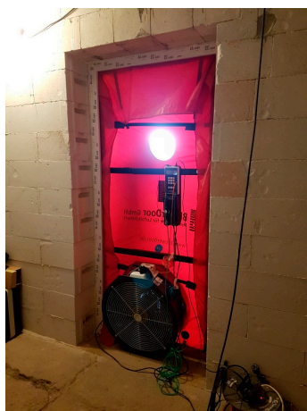
Figure 6. Blower door equipment installed and measurements of test chamber airtightness in progress.
