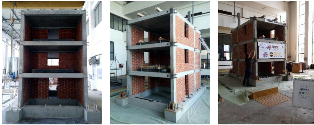
Figure 1. A view on the 1/2.5 scale three-story masonry infilled reinforced concrete frame building before testing
