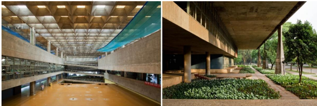
Figure 5. Vilanova Artigas - Architecture and Urbanism School, Sao Paulo (1961-1968)
