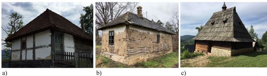
Fig. 9 Wooden building typology(W)—examples from Serbia: a a single-storey timber frame ( bondruk ) house close to Valjevo; b a single-storey rural house ( čatmara ) in the Nemenikuće village, and c a wood log rural house ( brvnara ), Zlatibor
