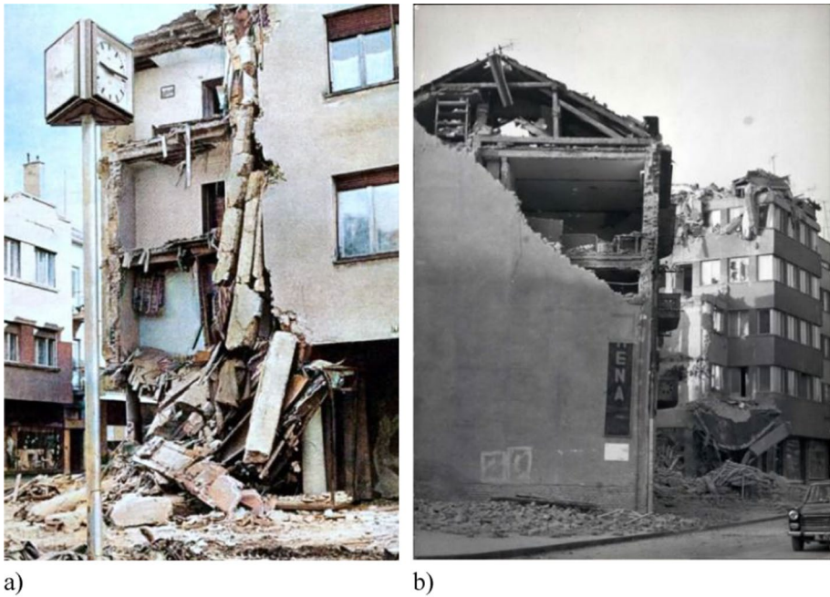
Fig. 21 Examples of type M2 residential URM buildings in Banja Luka affected by the 1969 earthquakes: a a partial collapse of the building with wooden floors (Banja Luka 2009) and b collapse of a gable wall (Blic 2019)
