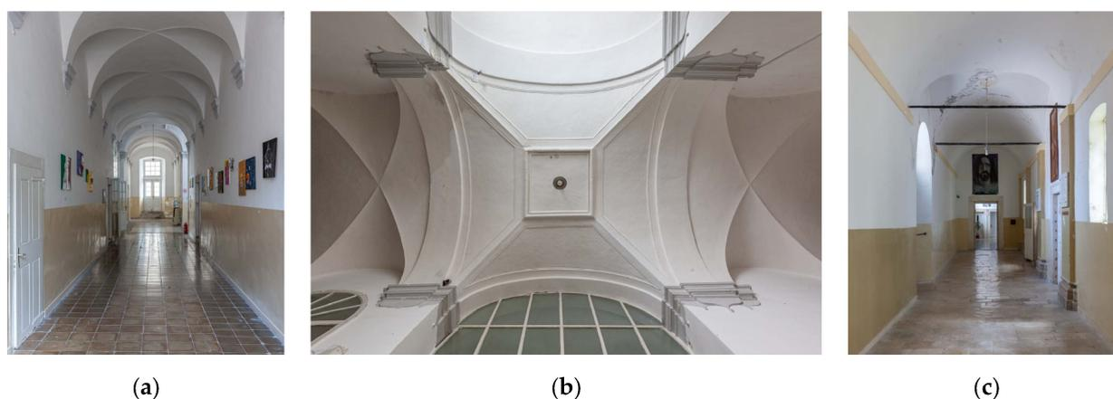
**Figure 4.** Different types of floor vaults: (a) Cross ribbed; (b) Intersection of different types of vaults; (c) Vaults reinforced with iron tie-rods (Photographic Collection of the Institute of Art History, Zagreb, photo by: Paolo Mofardin).
