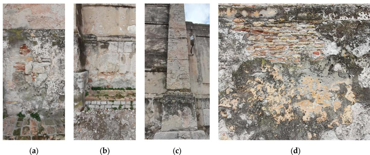
**Figure 3.** The non-uniform material composition of the external walls and columns: (a) wall with irregularly integrated bricks and stones; (b) wall with integrated layers of brick and stone on top of each other; (c) column brickwork; (d) exposed external wall portion made of bricks (illustration source: Davorin Penava).
