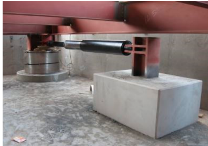
Figure 6. FVD's location in the isolated building [60].
