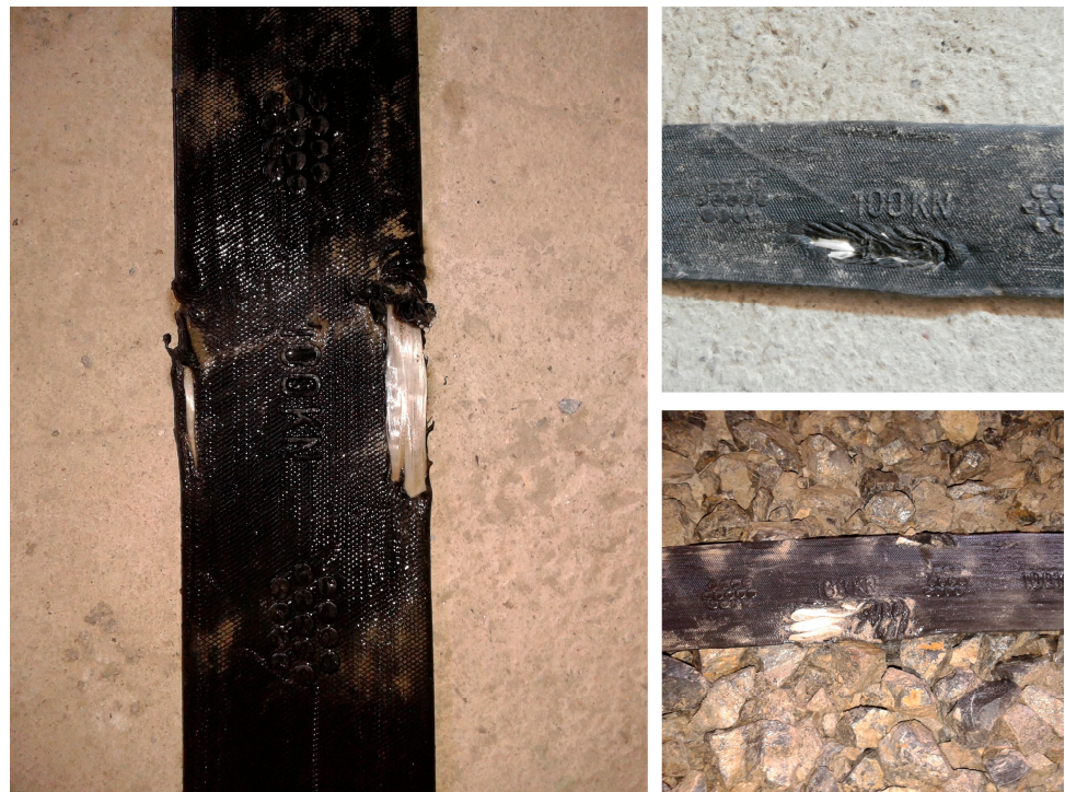
Figure 7. Damage of the straps in backfill material A.
