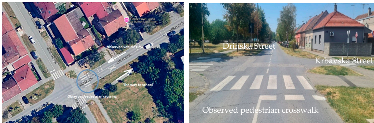
Figure 2. Observed pedestrian crosswalk [34].
