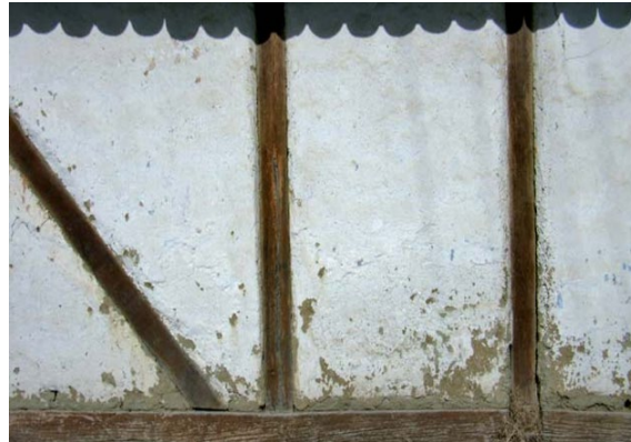
Figure 6. House walls constructed from wood and rammed earth or bricks, reinforced with wooden rope (bondruk). Reprinted with permission from ref. [3]. Copyright 2011 Lončar-Vicković, Stober.
