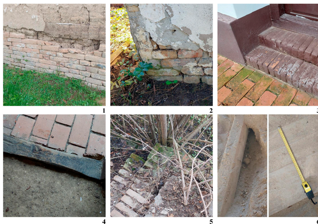
Figure 5. Various options for solving the houses plinths: (1)—RE with bricks cladding; (2)—brick plinth; (3)—dark brown colored brick plinth; (4)—RE floor; (5): brick stairs; (6)—wooden floors. Author's photos.
