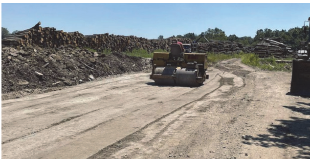
Figure 6. Compaction of the base course with wood ash
