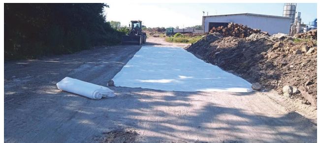
Figure 7. Geotextile on the base course with wood ash [32]
