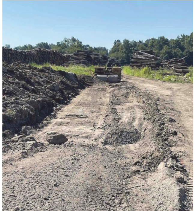
Figure 5. Filling of the base course with wood ash
