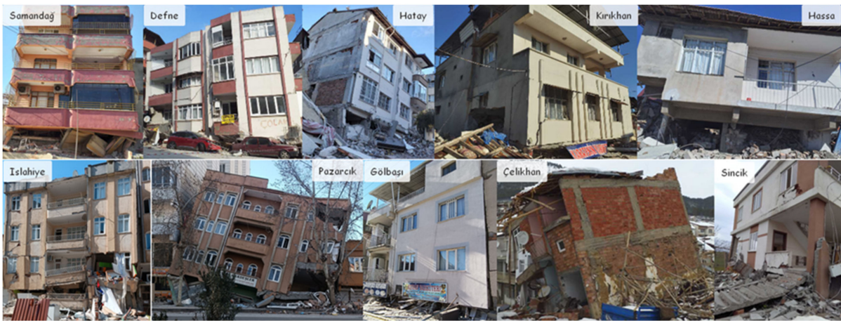
Figure 4. RC structures exposed to various levels of structural damage.
