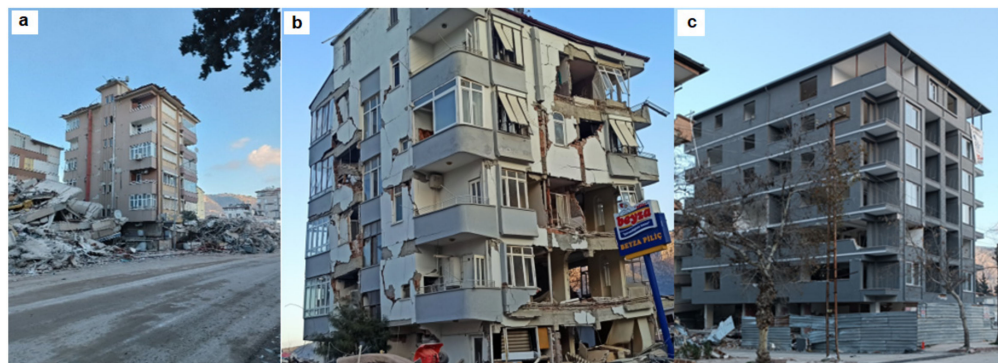
Figure 6. Examples of RC buildings with life safety ensured. (a) RC building standing despite the collapse of neighboring buildings, (b) example of RC building for pre-collapse performance level, and (c) example of a completed but not yet occupied building without damage.
