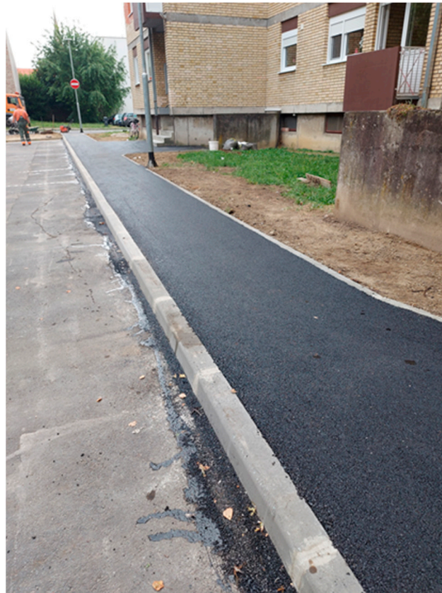
Figure 7. Completed test section.
