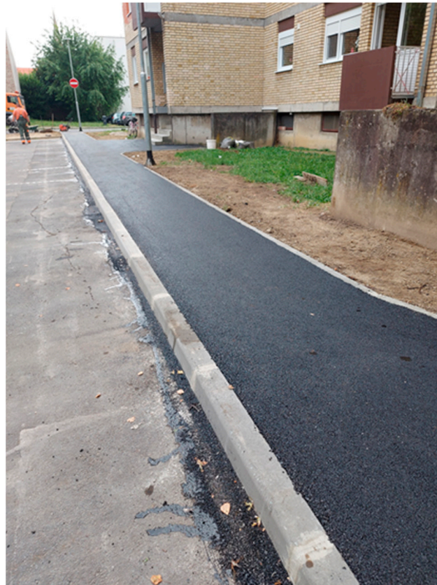
Figure 7. Completed test section.
