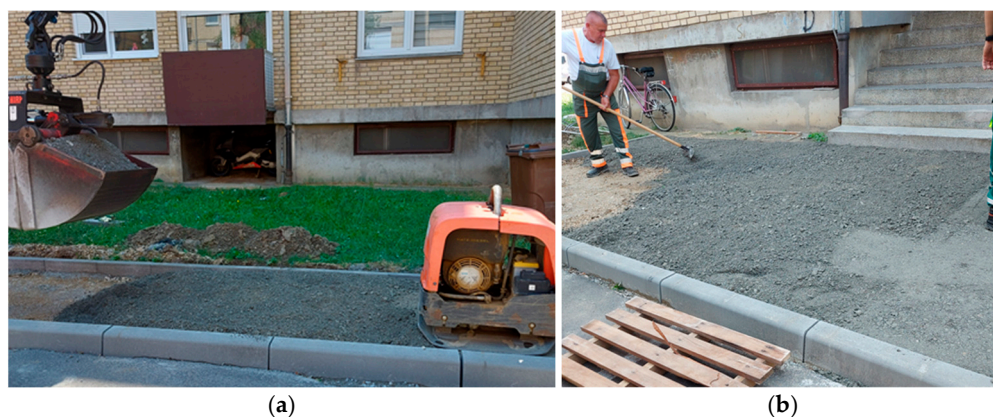
Figure 5. Cement-bound base layer construction: installation equipment (a) and manual spreading (b).
