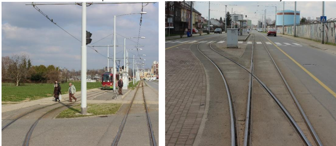
Figure 5 Passing loops with tram stops on Line 2
