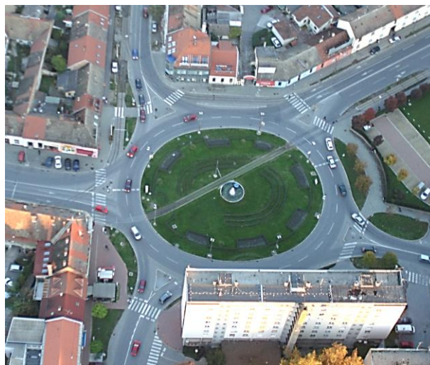
Figure 1 Aerial view of the Đakovština roundabout
