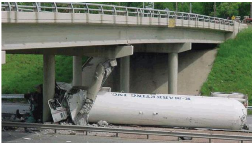
Figure 1 Impact between vehicle and column (U.S. highway) [8]
