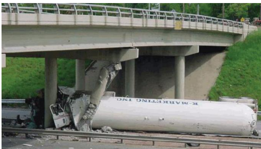
Figure 1 Impact between vehicle and column (U.S. highway) [8]
