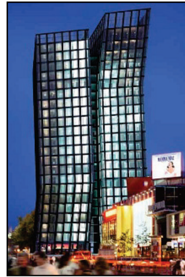
Figure 17 Commercial building in Hamburg (Germany) with an aluminium alloy curtain wall [41]
