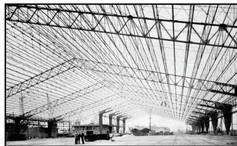
Figure 14 A frame system warehouse structure in Antwerpen [3]
