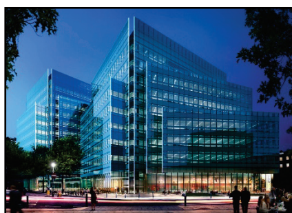
Figure 16 Office and building in London (England) with an aluminium alloy façade system [40]
