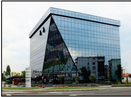
Figure 19 An office building with a structural silicone façade in Zagreb (Croatia) [43]
