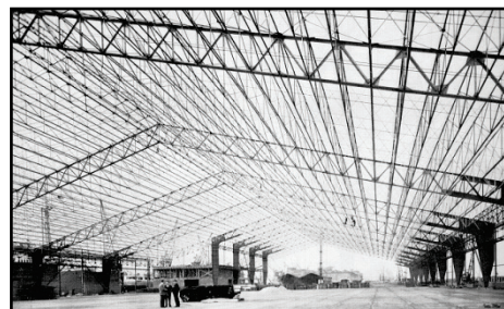
Figure 14 A frame system warehouse structure in Antwerpen [3]
