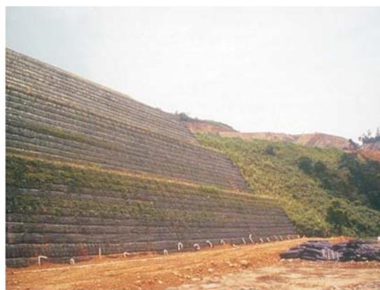
Figure 1 Reinforced soil embankment [7]
