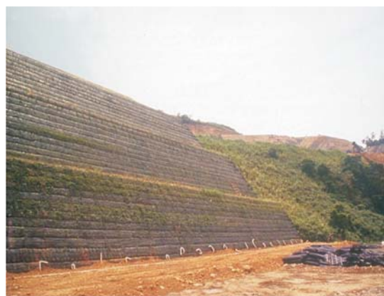
Figure 1 Reinforced soil embankment [7]
