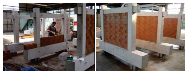
Figure 3 Construction of infill walls
