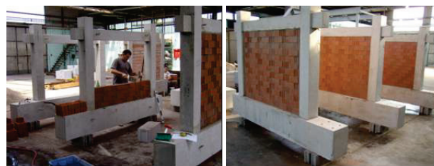
Figure 3 Construction of infill walls
