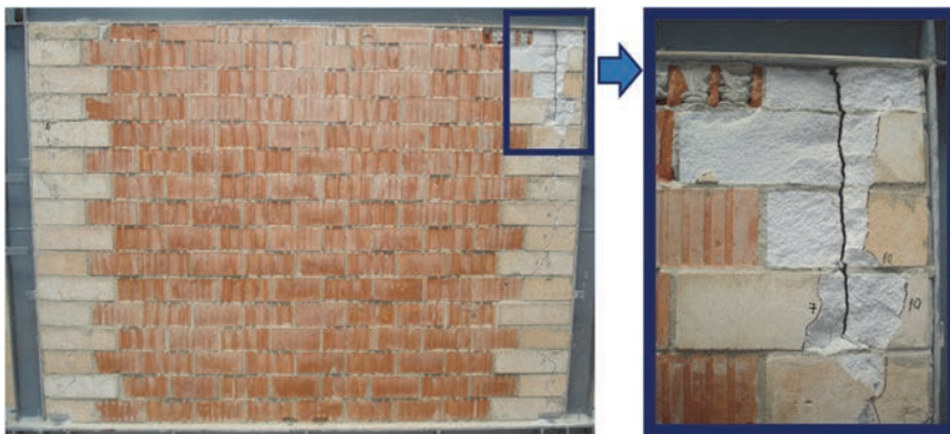
Figure 6. Photographs of specimen CA-1 after failure
