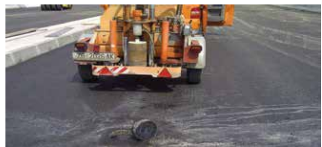
Figure 7. Sample taken at the Odra Viaduct from the completed waterproofing – asphalt system
